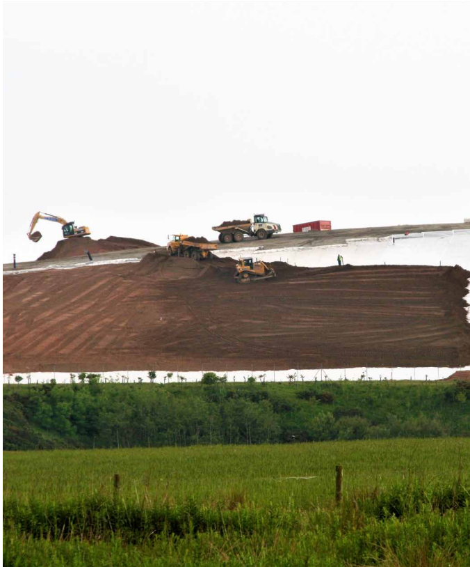
capping the landfill
